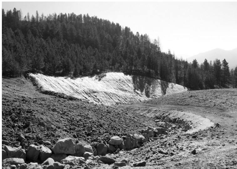
After: The open pit was filled in and Balarat Gulch, which used to flow into the pit, was diverted.
